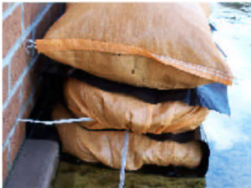
Proper sandbagging will create an “S” pattern. (See black material between sandbags)
